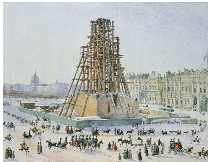
Prince Grigory Grigorievich Gagarin, Alexander Column in Scaffolding , The Hermitage, St. Petersburg (Figure 1)
